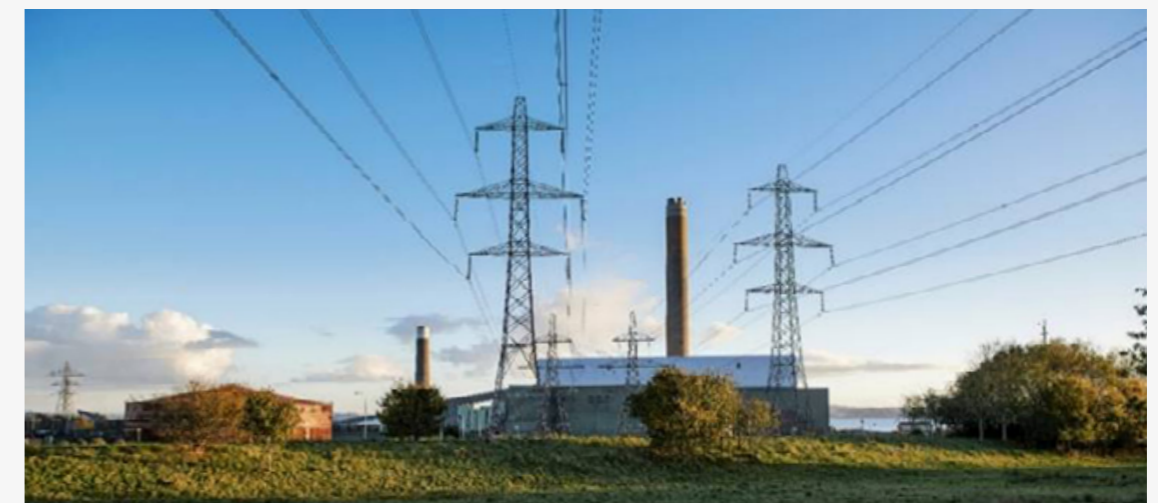
Picture 10: The EP Kilroot power station
